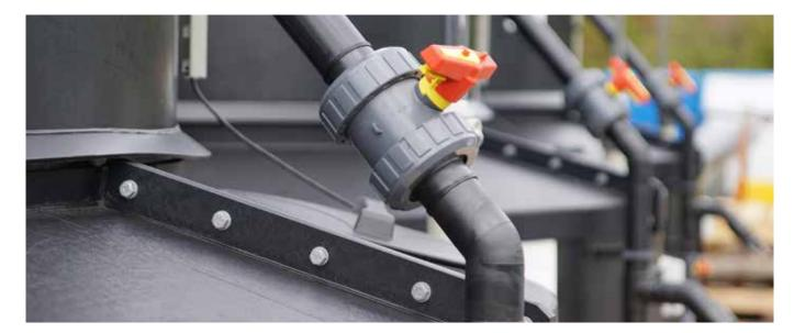
By contrast, excellent chemical and atmospheric corrosion resistance is offered by permanent bunds manufactured off-site using plastics like polyethylene (PE), polypropylene (PP) and polyvinyl chloride (PVC). For these, ensuring the appropriate strength is important (see 'Bund design issues').
